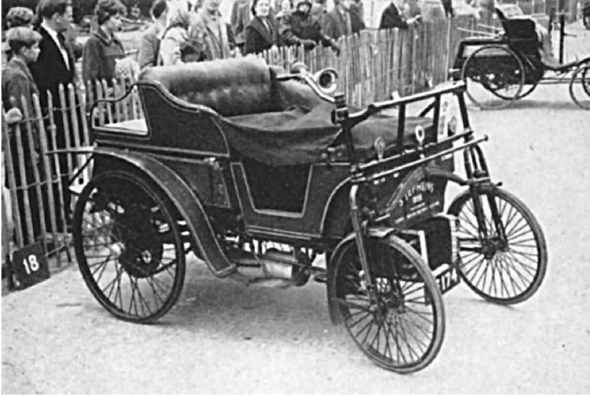
FIGURE 1.11. The vertical tubes suspension was probably introduced for the first time by Stephens in 1898.
